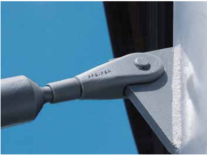
Approved compression rod connector
