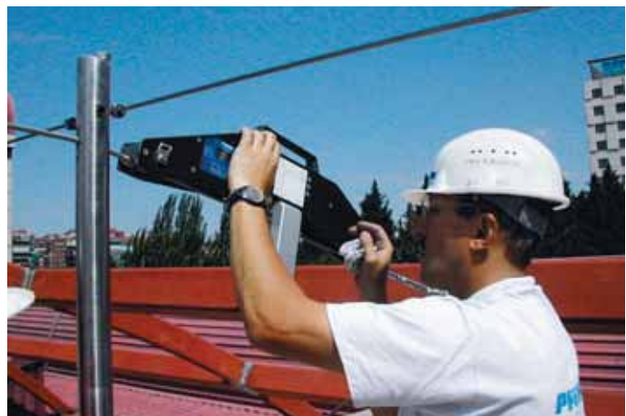
Measuring cable forces with a cable tension meter.
