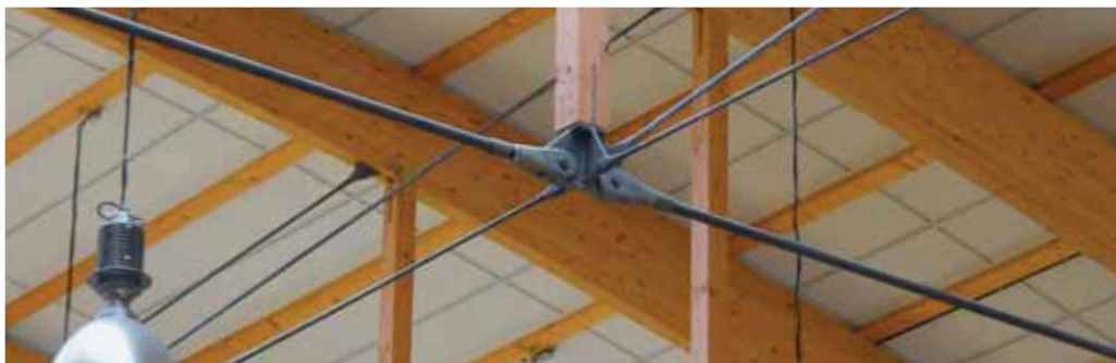
Ties in timber frame works
