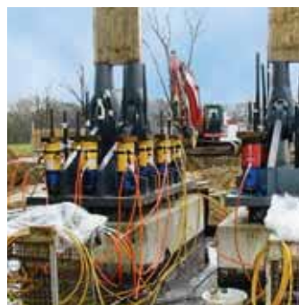
Pretensioning of a cable with hydraulic tensioning system
