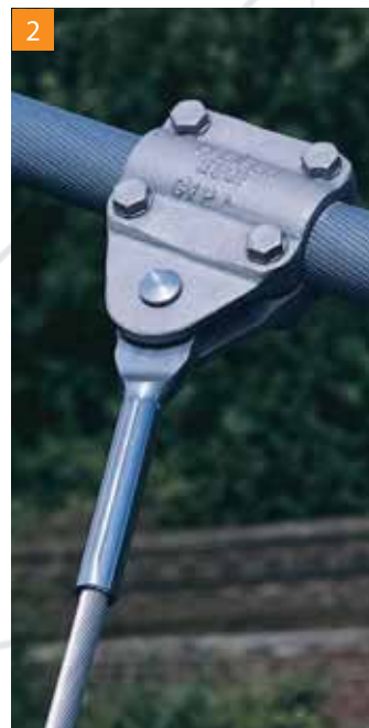
2 Connection hanger cable to suspension cable
