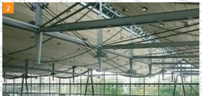
Inside view of main and secondary girders
