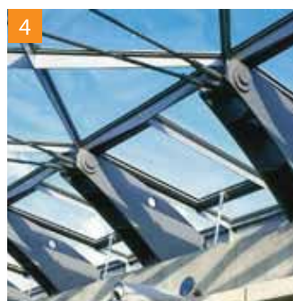
4 Connection stabilizing cable to frame
