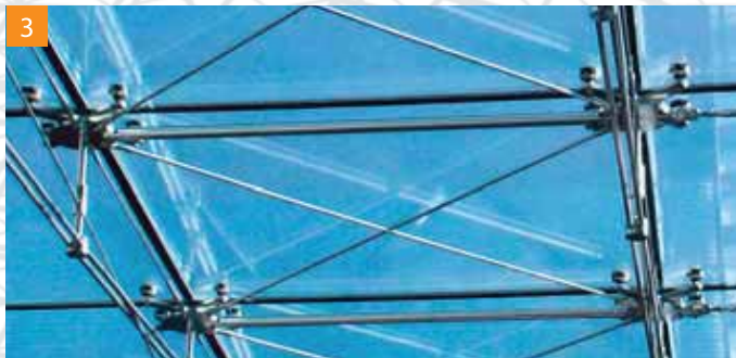
3 Connection compression strut to parallel cable net
