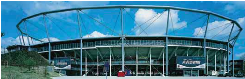
Bracings in the AWD Arena Hannover
