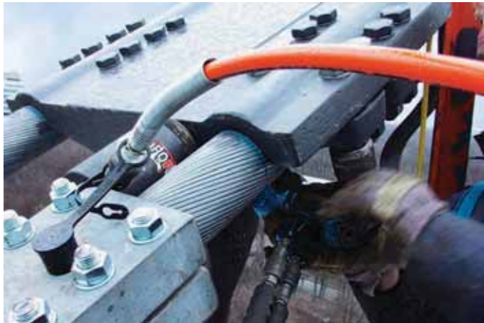
Precise prestressing, on a main cable and hanger construction.
