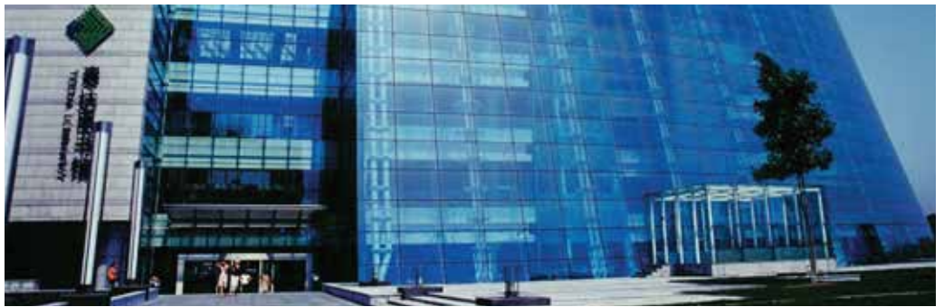
Curtain Walls, Roof Structures
