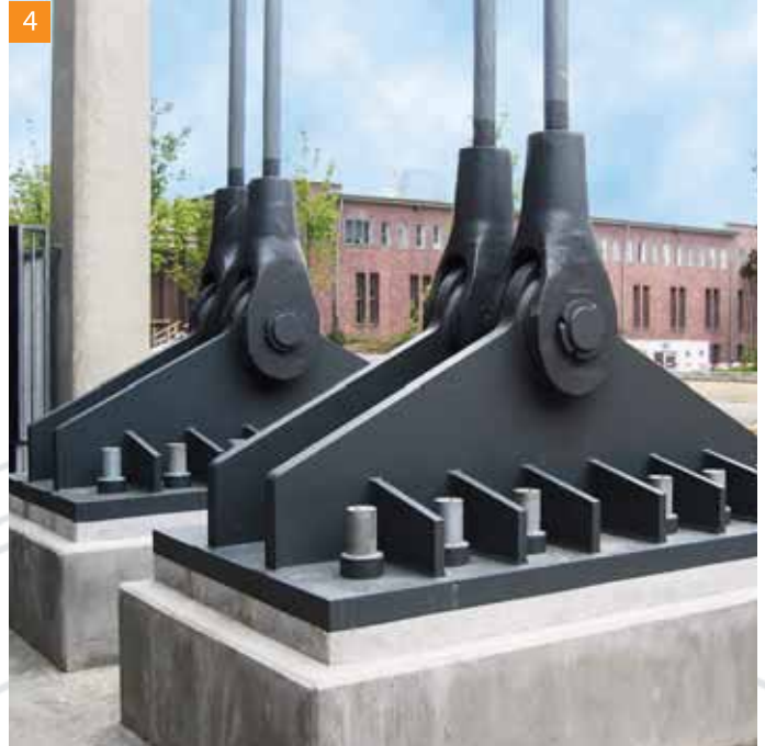
Connection stay cable to foundation
