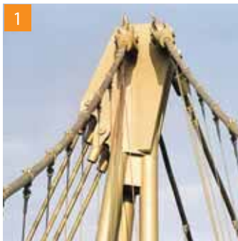
1 Connection suspension cable to pylon head with open spelter socket
